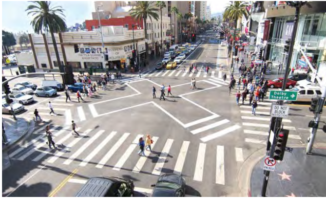
Pedestrian Scramble - Courtesy of LADOT (Los Angeles Department of Transport)
