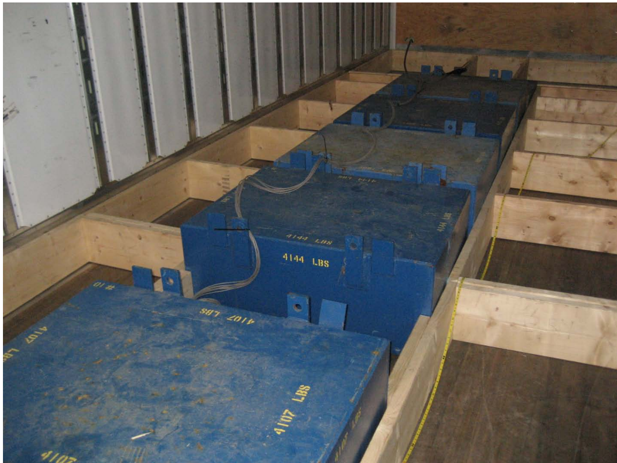
Figure 11: Ballast Installation
