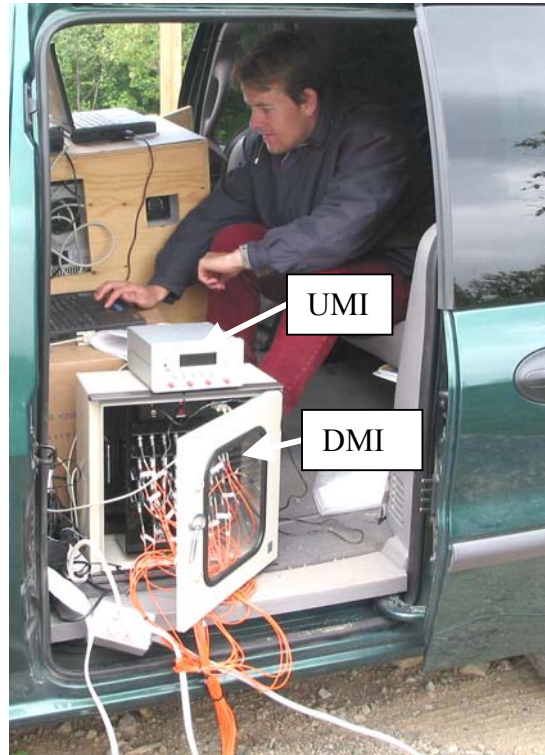
Figure 29 – Fibre-optic slab gauge data collection system
