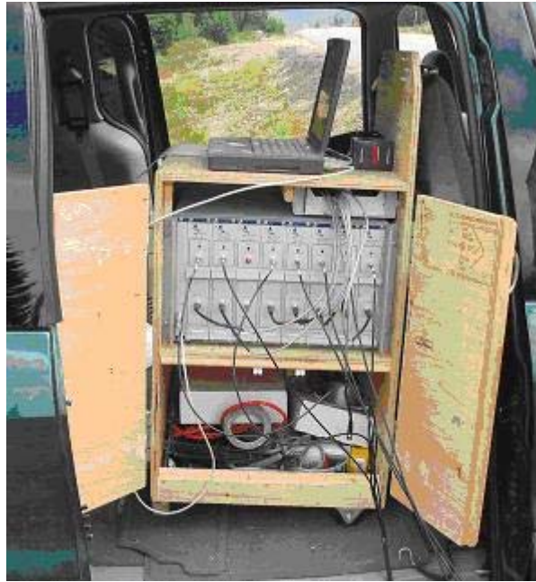
Figure 24 - Distortion gauge and multilevel deflectometer data collection system
