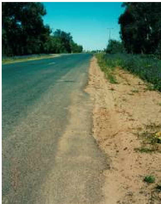
Figure 7.1: Poor road shoulder condition
