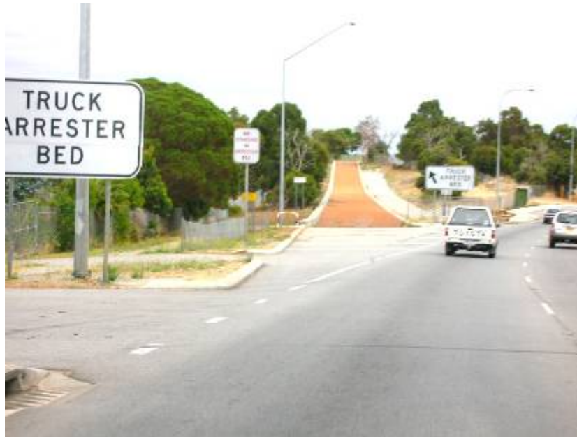
Figure 7.9: Truck arrester bed (Greenmount Hill, Perth)
