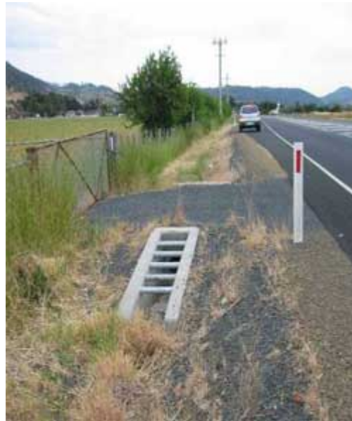
Figure 7.2: Driveable culvert
